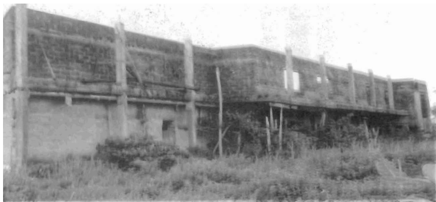
Photo 4: Abandoned Library Complex Building Project, Niger Delta University, Yenegoa.
